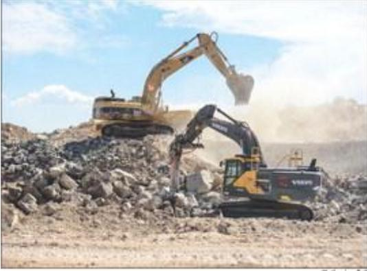
Rock blasting is underway at the Taos Regional Airport. Large boulders are crushed to a uniform size and reused.
